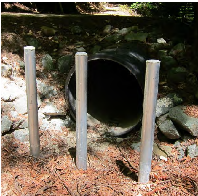
Left: Poles protect a culvert inlet from branches and sediment; Right: Culvert with rocks at outlet for energy dissipation
